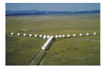
Very Large Array, New Mexico, USA. Y-shaped and nearly coplanar array of 27 25-m telescopes
