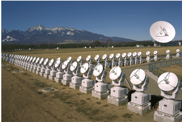
Nobeyama Radioheliograph (NoRH) antennas, Japan Observing frequencies 17 and 34 GHz
